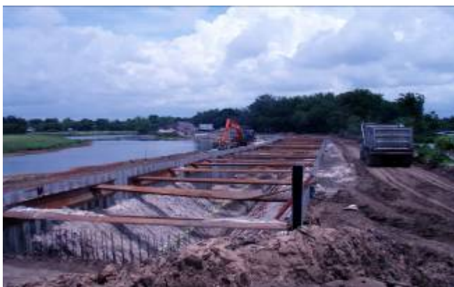
9. The bypass canal treatment trough during construction, looking east.
