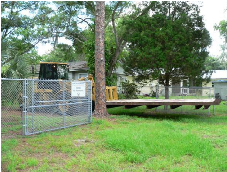
A bridge is placed over the ditch, allowing access to the uplands.
